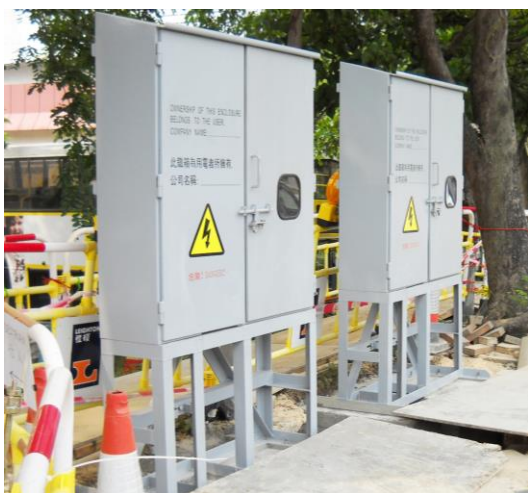
Weatherproof enclosures housing LV service cutout and meter supplied by HK Electric
