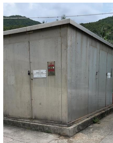
Pre-fabricated modular transformer pillars provided by HK Electric
